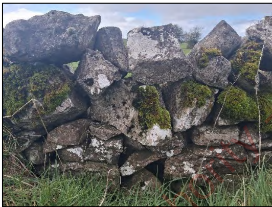
Plate 4-15 Section of stone wall proposed to be removed as part of the TDA works
