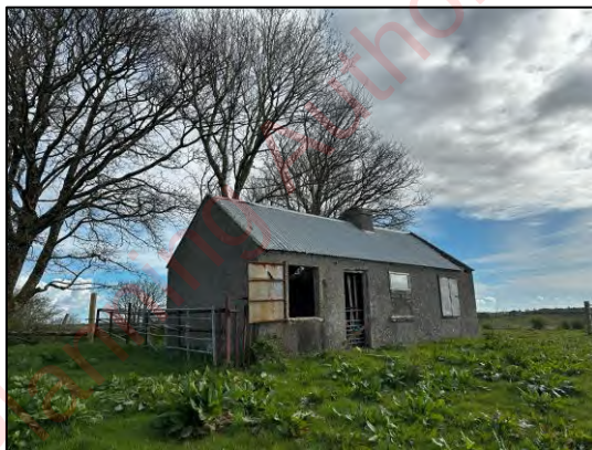
Plate 4-17 Southwest aspect of the farm shed (Structure 1) showing the concrete exterior, corrugated iron roof, and surrounding habitat.
