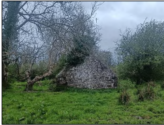
Plate 3-1 Northeast aspect of Structure No. 3
