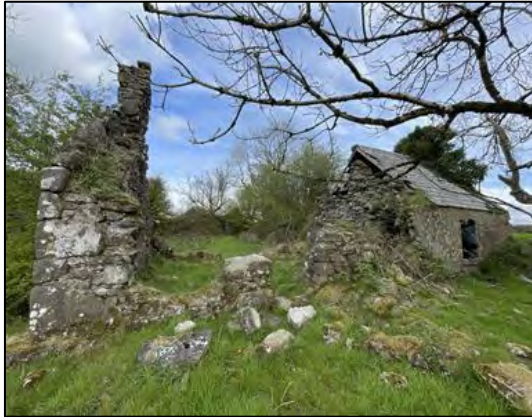
Plate 4-22 Southwest aspect of Structure 2 showing the exterior stone structure, slate roof, & surrounding habitat.
