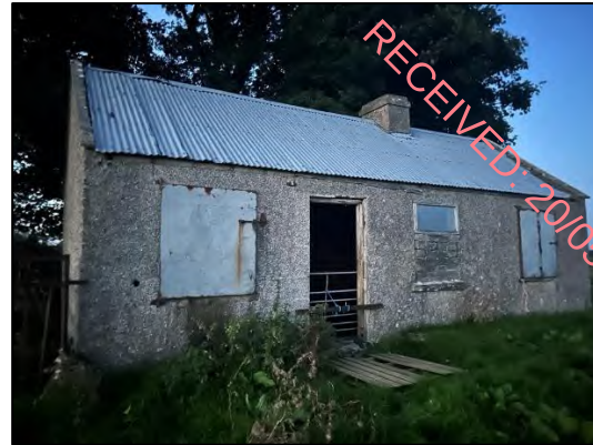
Plate 3-2 Southern aspect of Structure No. 1
